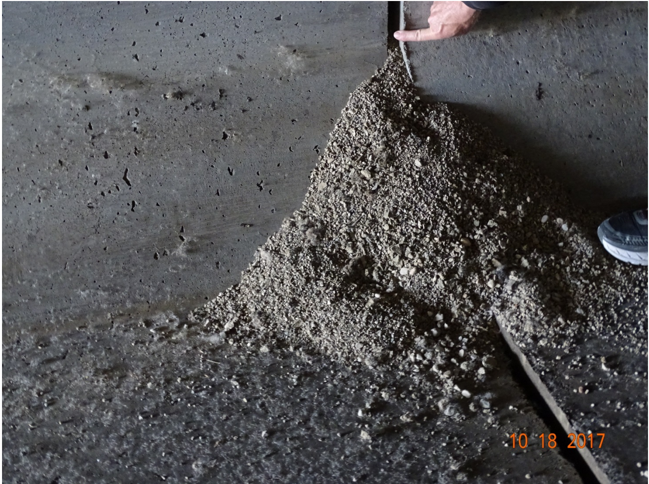
Photo taken inside the conduit showing sand leaking from the joint. A few other joints had sand leaking.
