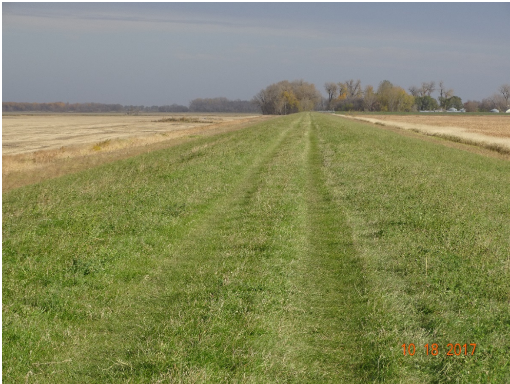
Photo taken near the southwest corner of the dam. The grass cover on the embankment is in good condition.
